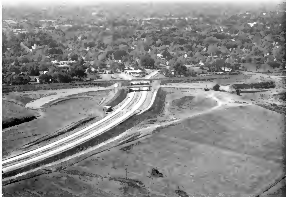
"A" Street Overcrossing and floodgates are shown in center foreground with Southern Pacific Railroad line immediately in back of these structures. View is looking south toward Sacramento.
